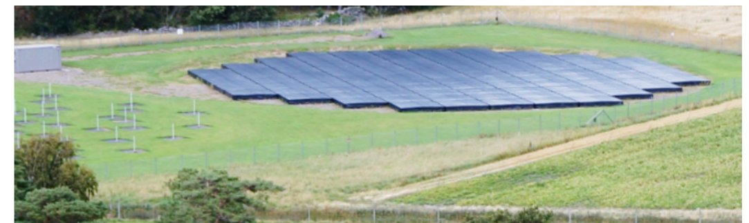
LOFAR station in Onsala. Credits: Onsala Space Observatory/R. Hammargren
