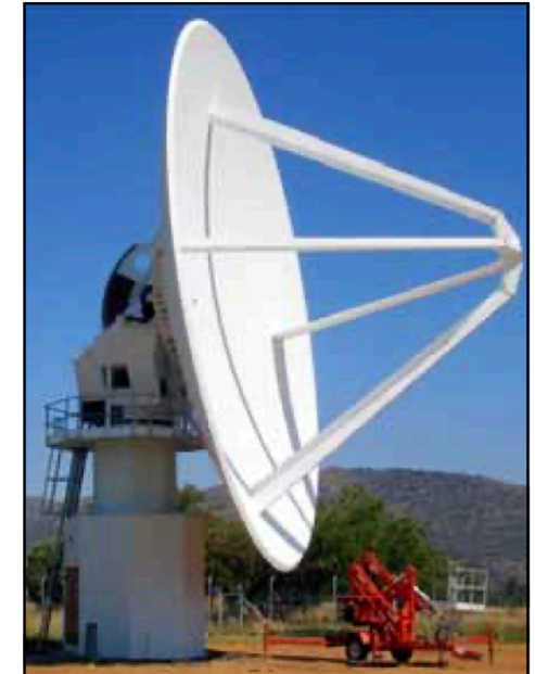
The meerKAT prototype with all major mechanical components installed. The prototype is at the Hartebeesthoek Radio Astronomy Observatory in South Africa.
