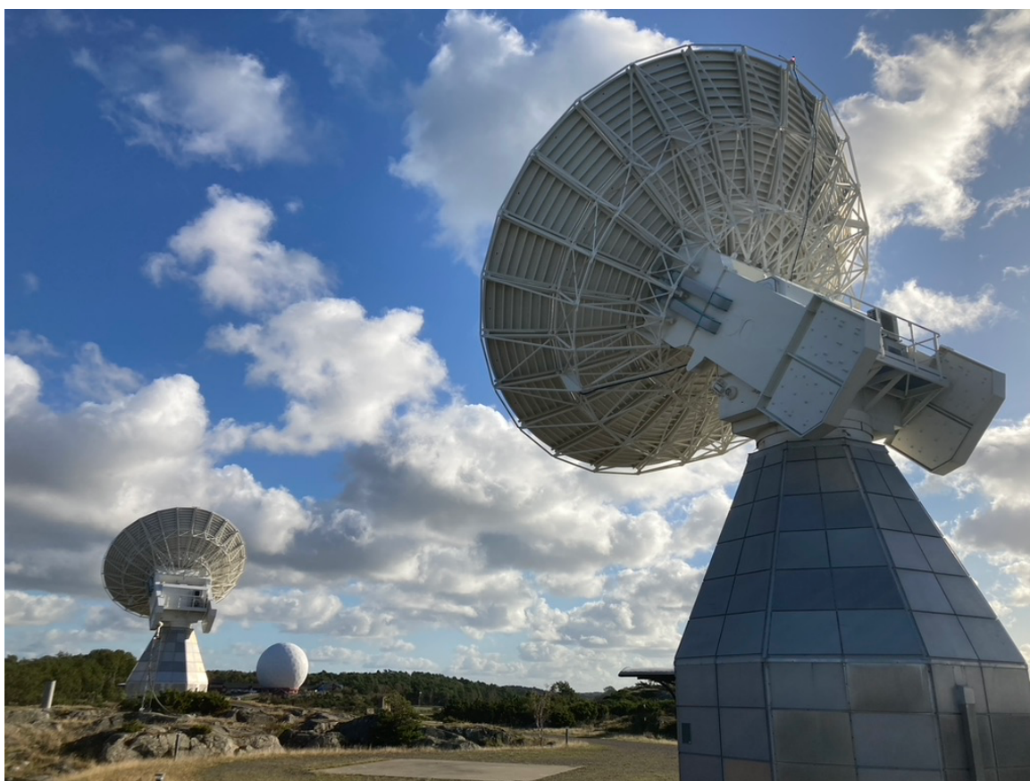
Figure 1: Telescopes at the Onsala Space Observatory that are used for geodetic VLBI observations: the 20 m telescope (middle) and the twin telescopes (left and right).
