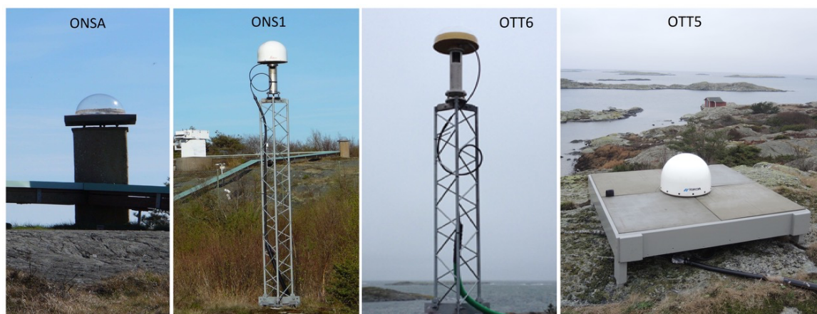
Figure 3: Some of the GNSS installations at OSO.
